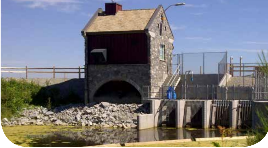
The new Maple Drainage Pump Station in Crescent Beach improves drainage and reduces the risk of flooding.
